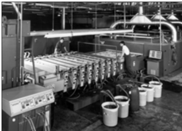
Figure 2.10 Rotary-screen printing machine (Stork BV)
